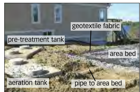
Pre-treatment tank followed by an aeration tank and area bed.
